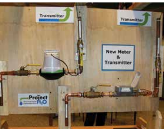
This mock up was used to show consumers what the meter would look like in their homes, and how the new meter installation compared with that currently in place.
