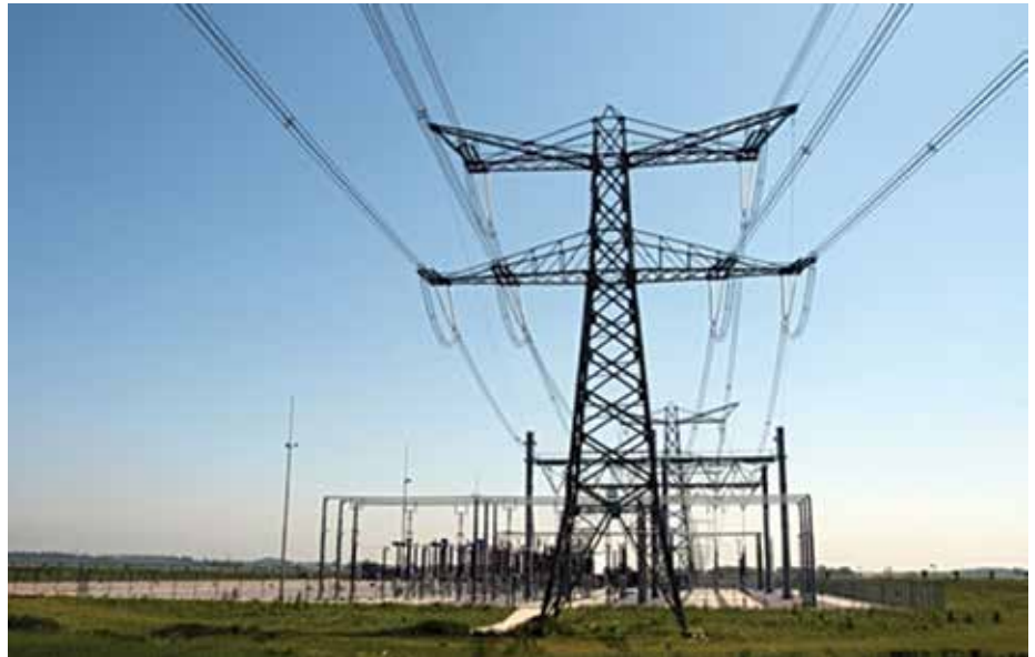
In the Infrac 10 kV distribution network each 10/0.4kV transformer substation is guarded and monitored.
